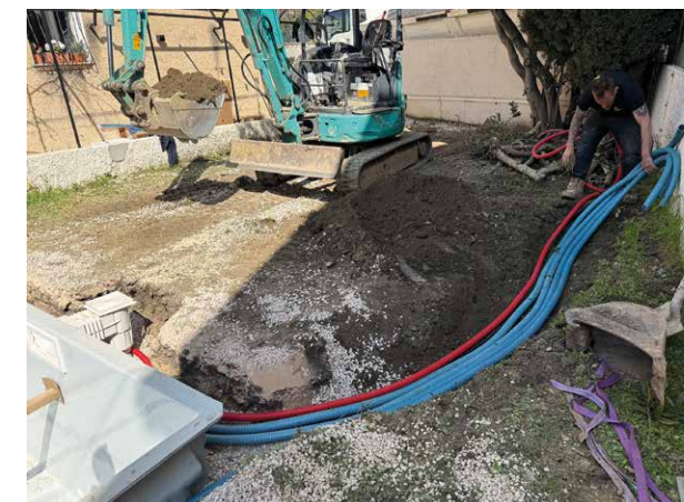
8/ Raccordements hydrauliques
